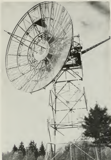
From this 40-foot antenna at Covey Hill, Quebec, UHF signals are sent without relays to RCA's laboratory at Riverhead, L. I., by scatter propagation.
